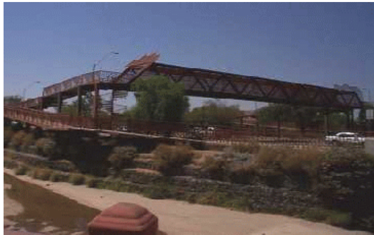
Figure 15. Grade-separated crossings are sometimes used when other measures are not feasible to provide safe pedestrian crossings.
