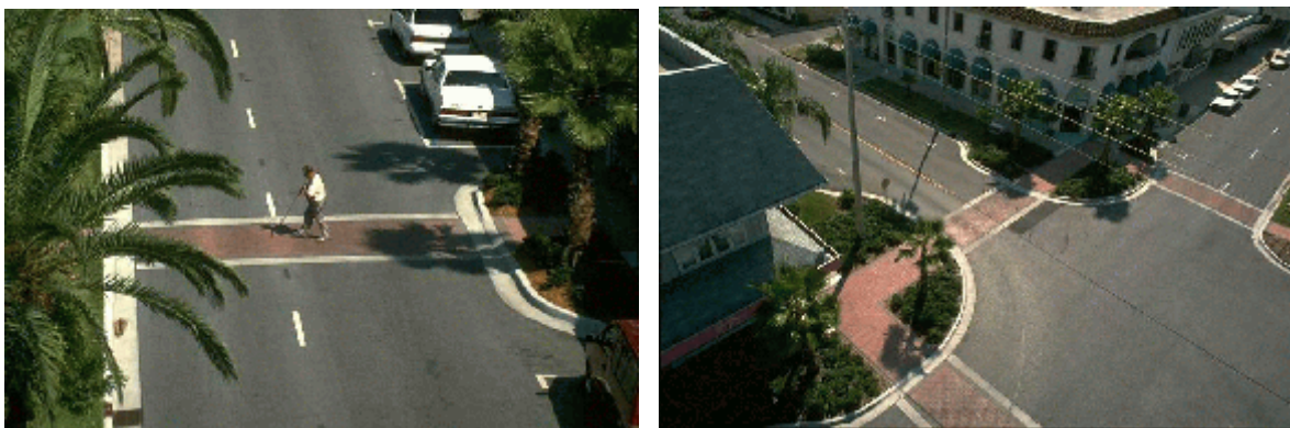
Figure 12. Curb extensions at intersections or midblock locations will shorten the crossing distance for pedestrians.
